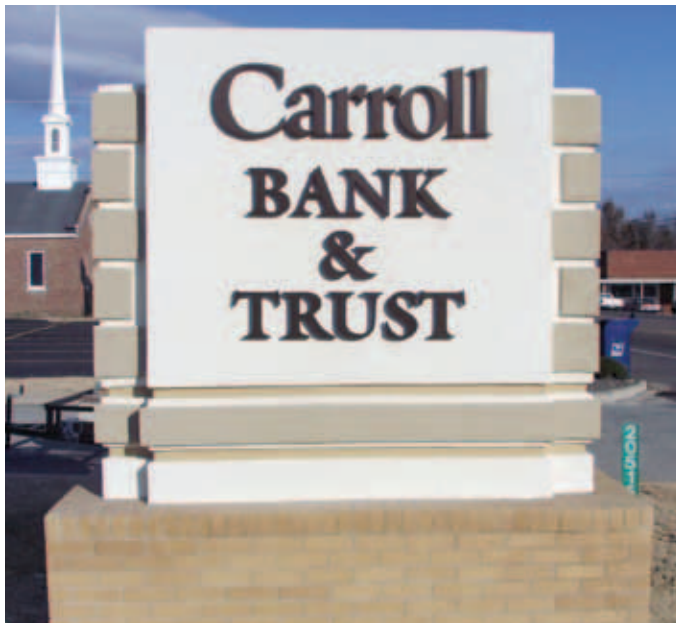
52-by-60-in. double-faced EIFS monument with water-jet cut Gemini letters ( www.signletters.com ); pedestal and monument provided by builder
