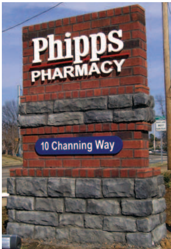
CNC-cut PVC letters and graphics finished with acrylic latex paint
