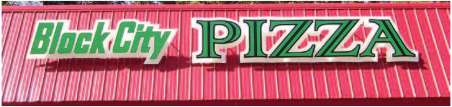
3-by-32-ft. LED backlit sign; letters are cut from 2-in. EPS foam and coated with Chem-Coat 2538 two-part urethane. Backs of letters are routed out to provide a space for the low-voltage high-output LED lamps. The letters are mounted 2-in. off the aluminum composite material surface, which is painted flat white to amplify the halo effect at night.
